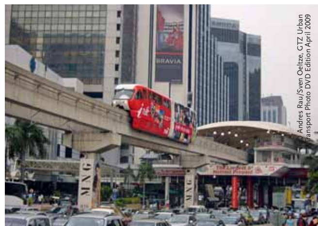
FIGURE 4: ... or light rail transit (Kuala Lumpur, Malaysia) show a strong interest among local stakeholders to improve transport systems.
